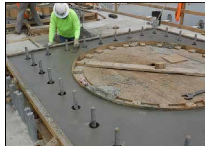
JCC1 Concrete placement for pump sole plate
