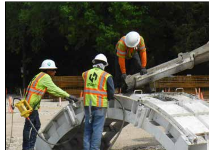
PL17TUN Casting concrete tunnel liner segment
