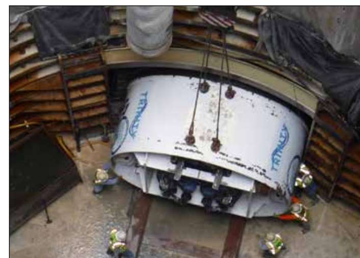
PL17TUN Cutter head of Tunnel Bore Machine set in access shaft
